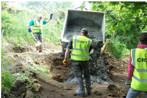
Bridge foundations on Rodanbraes
